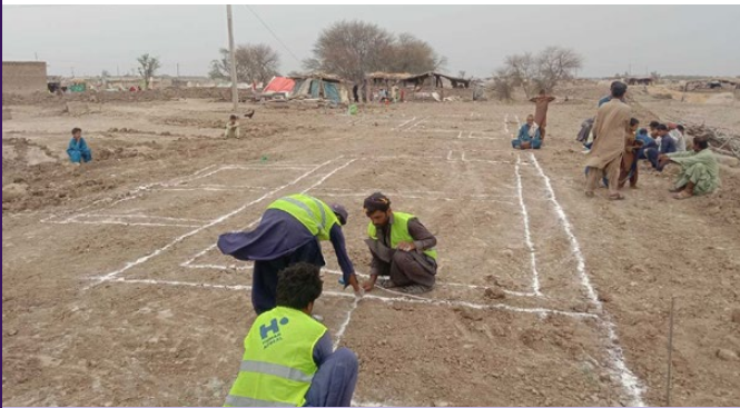
The positions of houses being marked out in the village.
