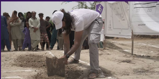
Ground being broken at the new housing project.
