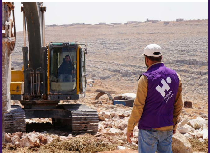
Human Appeal staff watching construction begin.
