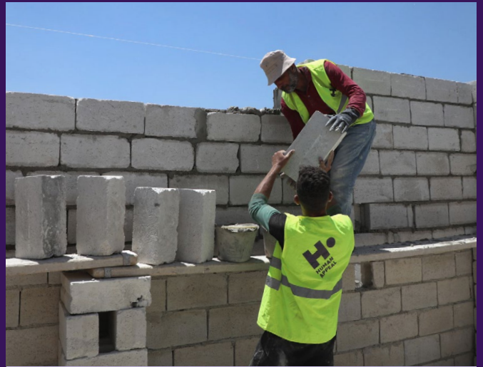
Homes being constructed in Al-Yasameen Village.
